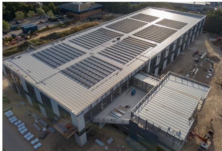
Aerial view of the building under construction
