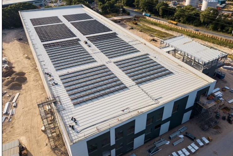
High angle view of the building under construction
