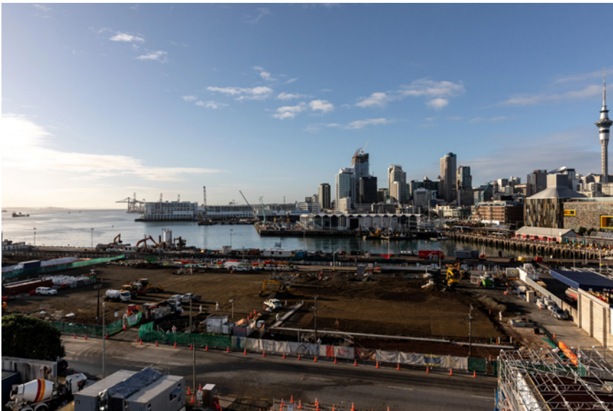
The silos have gone - making way for challenger bases on Wynyard Wharf, to be handed over to teams in August. Photo: WEA © Emirates Team New Zealand
